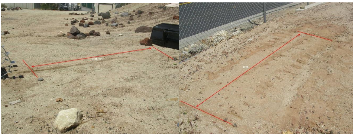
Figure 3: Track 2 (left) and Track 3 (right). Note that Tracks 1, 2 and 4 were constructed in the same general vicinity so their soil properties were similar.
